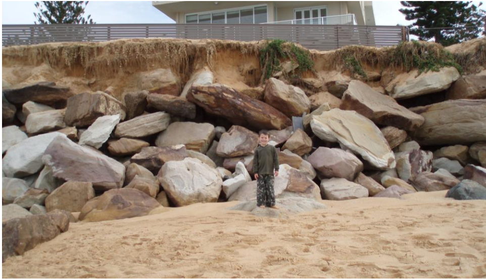
Figure 2: Exposed Rock Protection at Narrabeen Beach in July 2007
